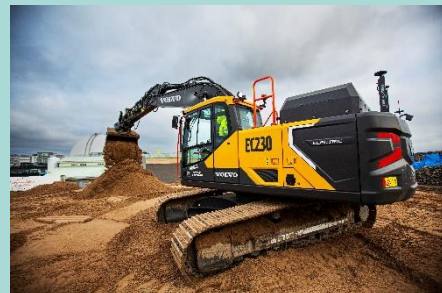
Foto: Volvo Construction Equipment
