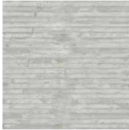
Betong, gjuten i brädform
