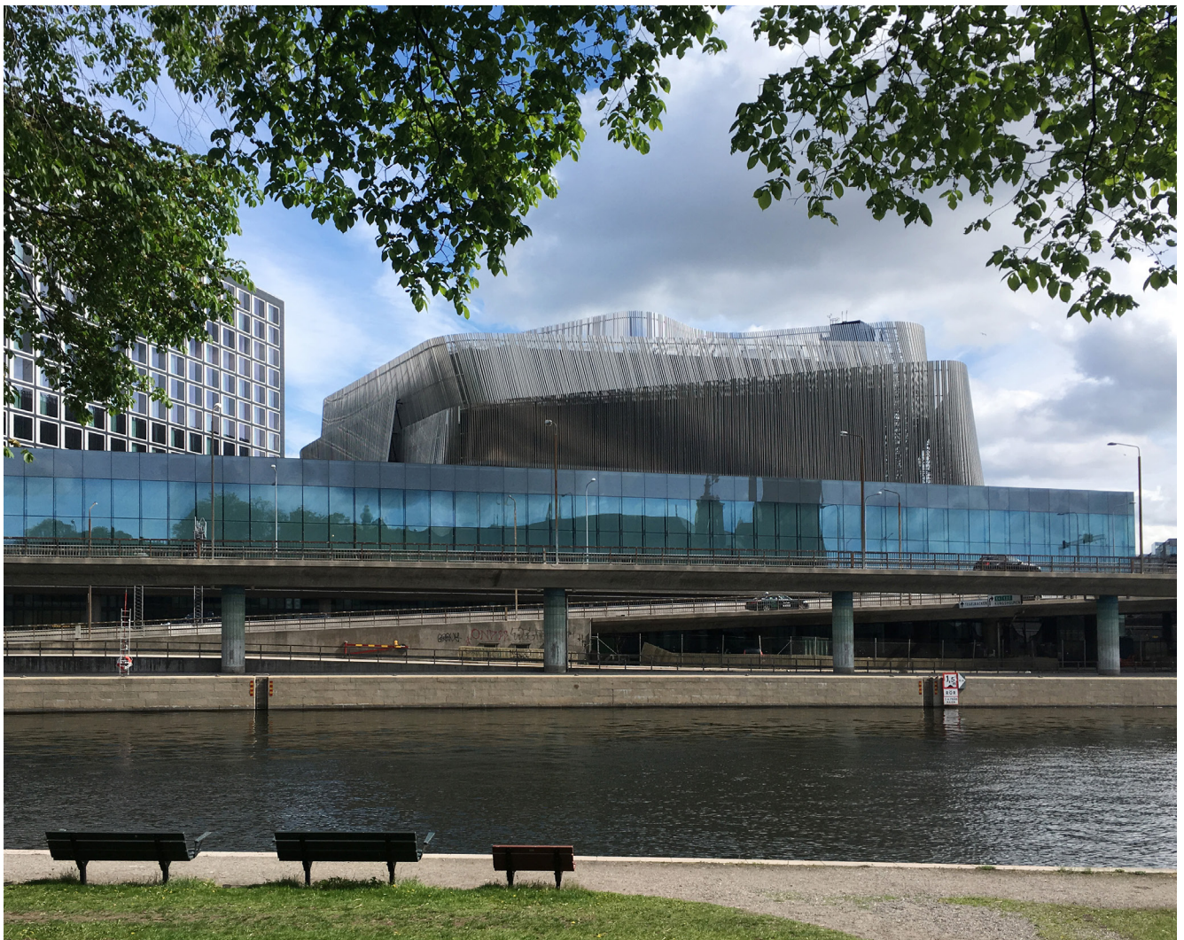
Exempel glasfasad, Stockholm city.
