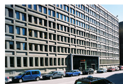
8. Trollhättan 29, Statens investeringsbank 1973-75, Boijesen & Efvergren. Foto: Göran Fredriksson SSM.
