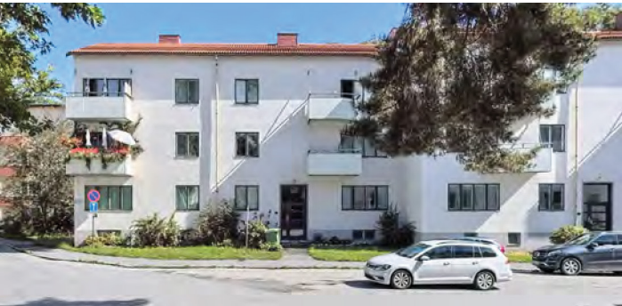
FASADMATERIAL LJUS PUTS
