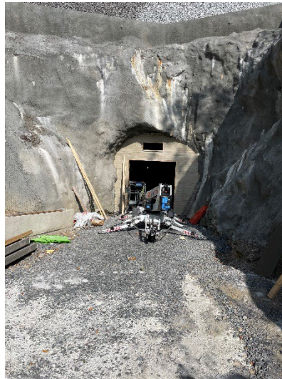
Tunnel under pågående renovering.
